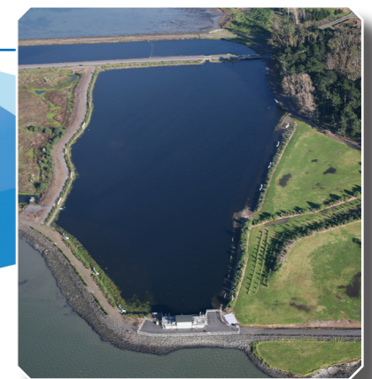
After filtration the treated water flows along a distribution channel to a storage basin. This water is pumped out twice daily at high tide into the Manukau Harbour.
