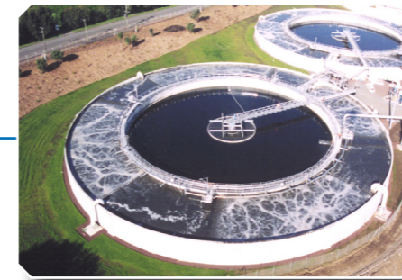
One of the nine reactor clarifiers
