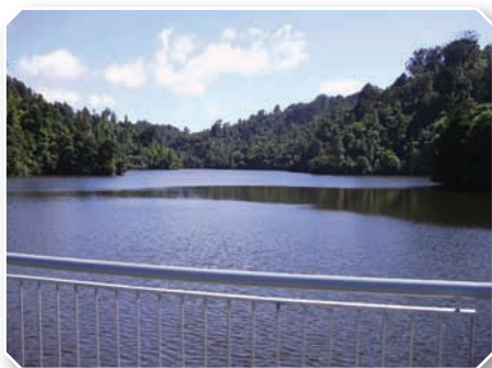
The spectacular Upper Nihotupu Dam reservoir.
