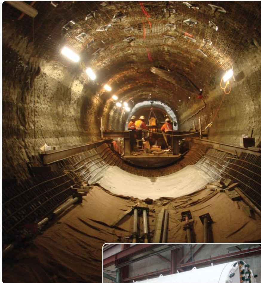
The tunnel between the temporary and permanent shafts is completed in preparation for the TBM's arrival (above).
