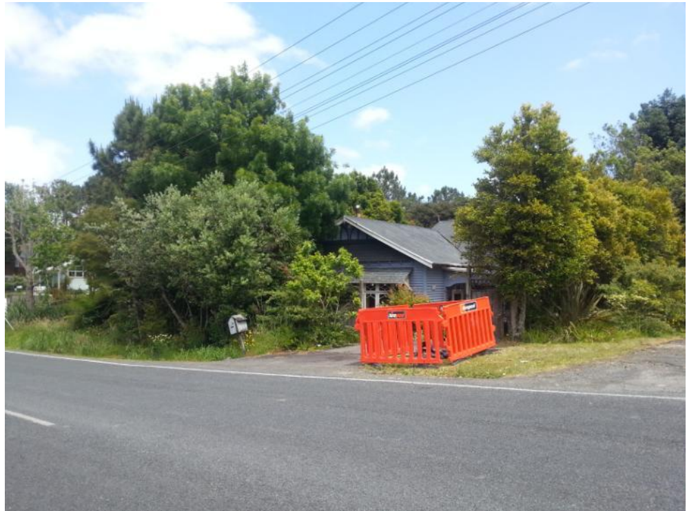
Figure 21. CHI 3729, 262 Glengarry Road.
