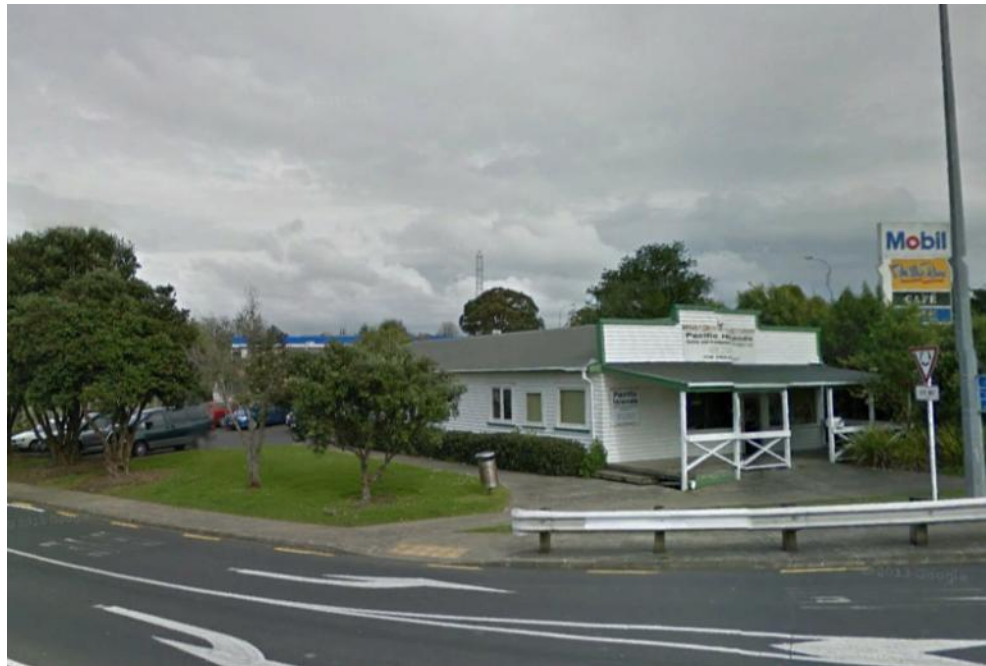
Figure 22. Looking south towards CHI 3804 – former Massey Post Office
